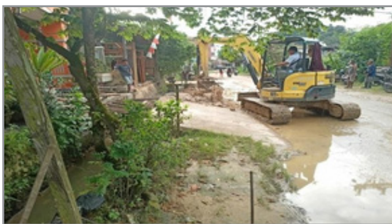
Figure2: Excavation of Drainage Channels.
