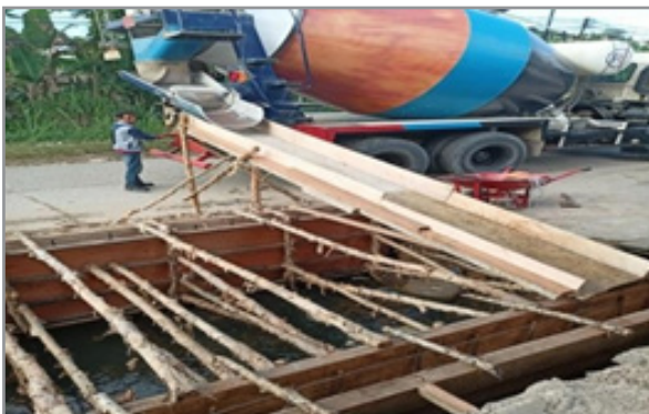
Figure 6: Concrete Overlay.
