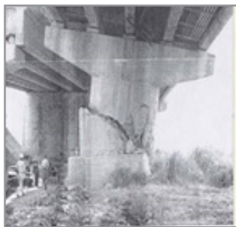
Figure 2: Failure of bridge pier during CHI-CHI, Taiwan earthquake, 1999
