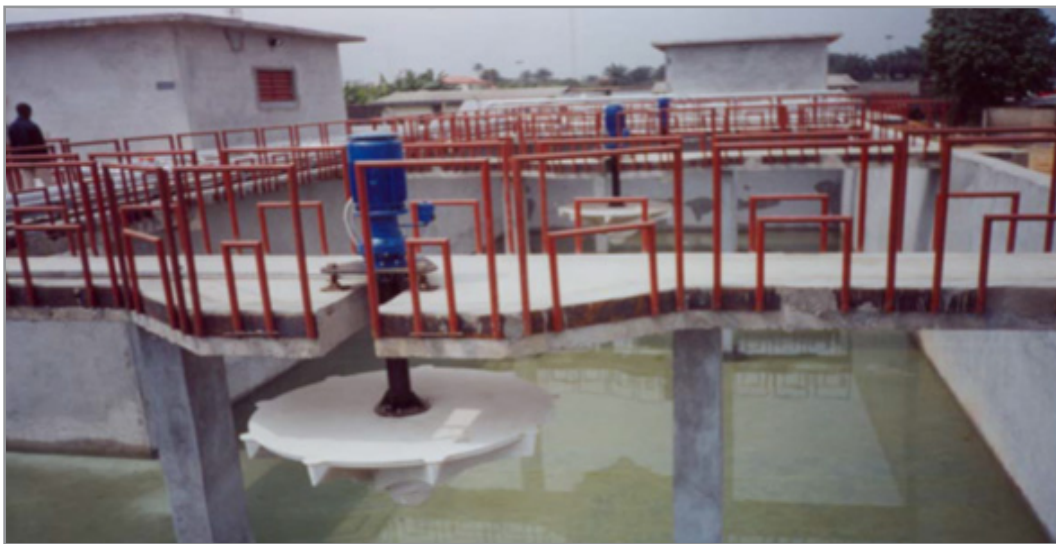
Plate 2: Aerobic Waste Water Treatment
