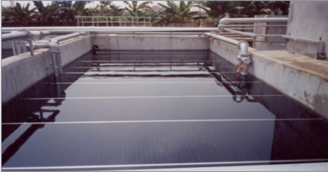
Plate 1: Rectangular Waste Water Sedimentation Tank
