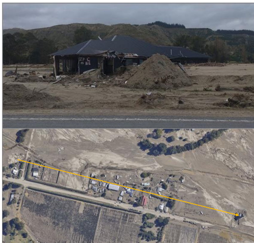
Figure 5: Photo A Shows the Relocated house. Photo B Shows the Original Location at the Top Left of the Image and where it Travelled to Approximately 650 m Downriver.
