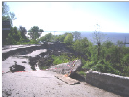
Figure 1: Sliding of the roadbed in Ulyanovsk due to inefficient drainage and increased vibration from the railway transport and heavy vehicles.
